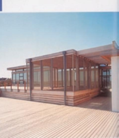
The new construction uses as a reference –in terms of formal language and structural system– the old house that occupied the lot and to which the new one is attached. The addition is lightly separated from the original building, yet the two are united by a wooden roof, which respects the existing architecture.
